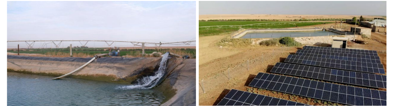
75kW Solar Irrigation Project in Morocco
